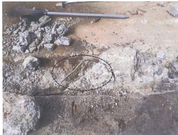
Photo. 9 Remains of a rebar in the concrete wall
